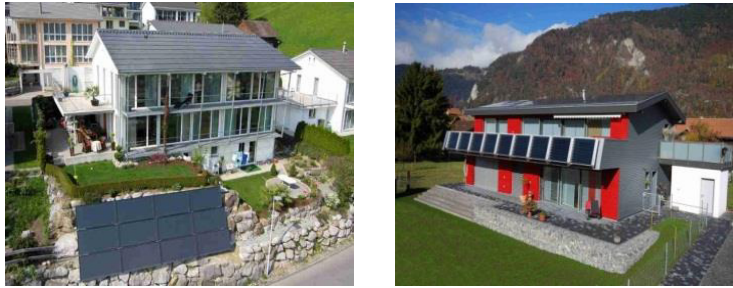
Fig. 5. On-site generation (pictures [2]).
