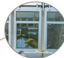
Fenster Orion, Zürich
