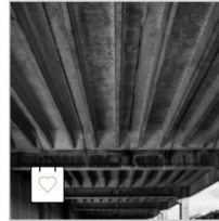
Rippenplatte Stahlbeton / L=5.99m,B=1.495m
