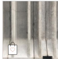
Rippenplatte Stahlbeton / L=10.39m,B=1.495m
