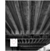
Rippenplatte Stahlbeton / L=8.97m,B=1.495m
