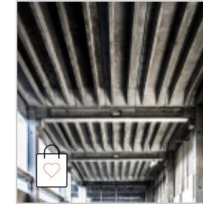
Rippenplatte Stahlbeton / L=6.84m,B=1.495m
